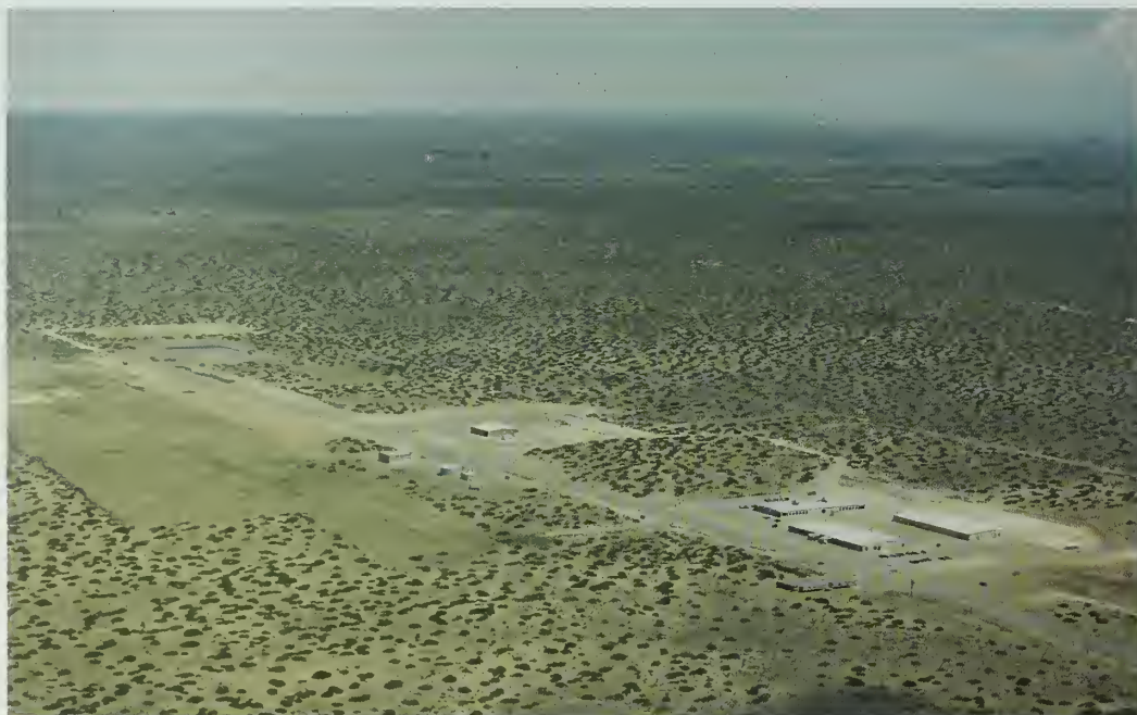
Fig. 3-17. A special facility for the Ground-Based Laser project was constructed at the White Sands Missile Range.
